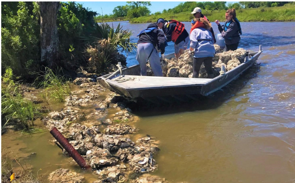
Figure 18: Volunteers add recycled oyster shells to an artificial reef in Pointe-aux-Chenes (Coalition to Restore Coastal Louisiana, 2019).
