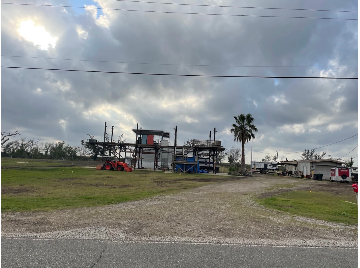
Figure 21: A home on Pointe-aux-Chenes road after Hurricane Ida
