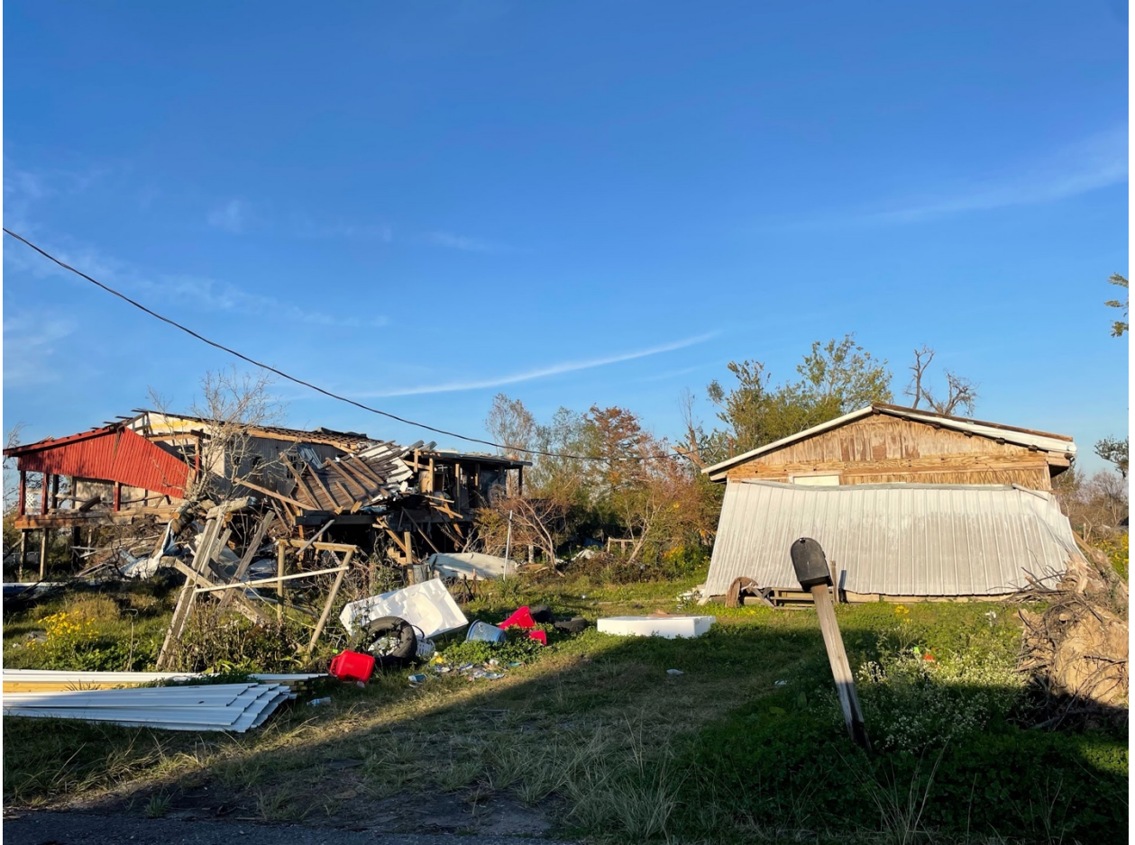
Figure 13: Homes destroyed by Hurricane Ida
