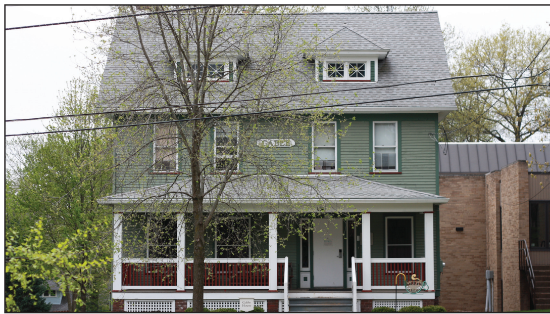
Above, Gable House, which underwent repairs and has been cleared to host Common Grounds events in their home (Photo by Mel Griffith).
