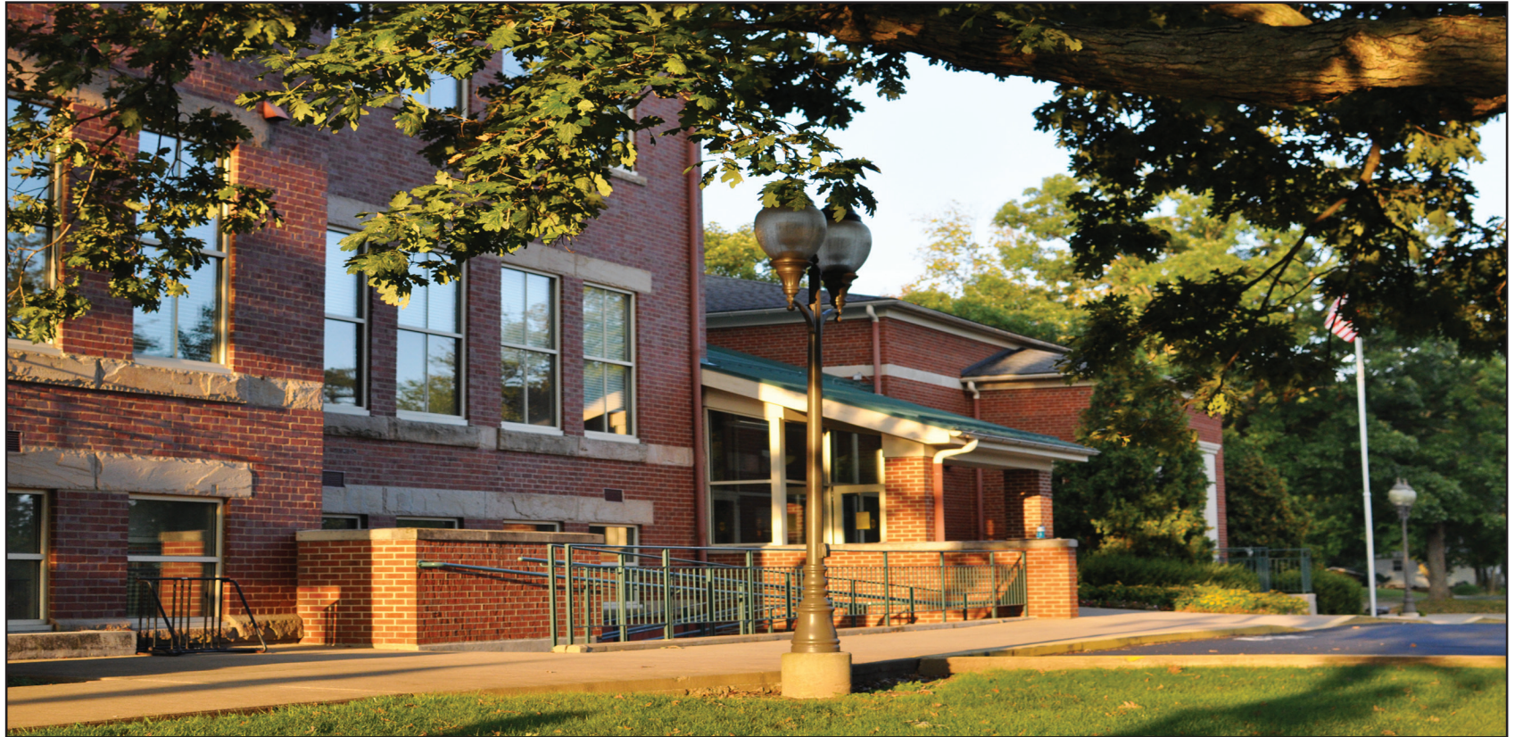
The Gault Schoolhouse is in the process of being renovated as it is turned into Wooster's newest residence hall. Students had the opportunity to see a mockup single on Sept. 18 (Photo by Ian Benson).
