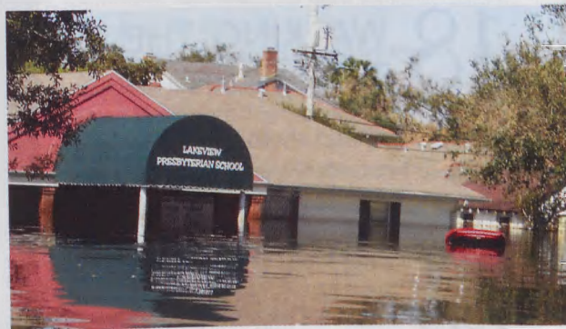
Broken levees after Hurricane Katrina flooded Lakeview Presbyterian School and its New Orleans neighborhood.
